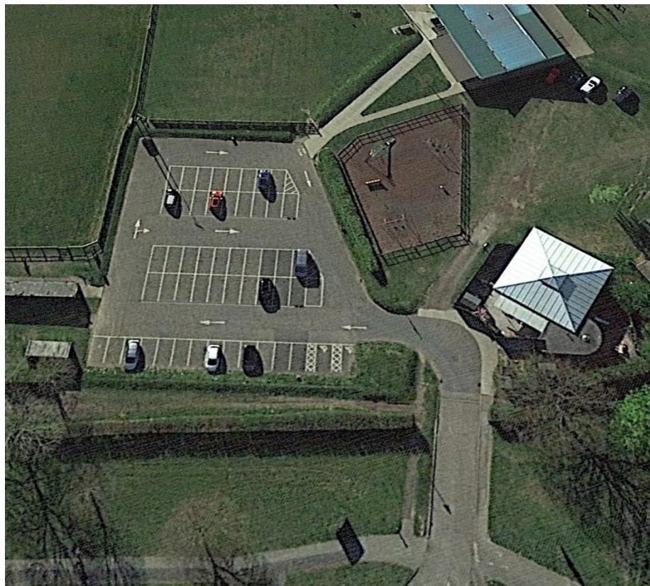
figure 50: The Existing Chilton Fields Car Park
