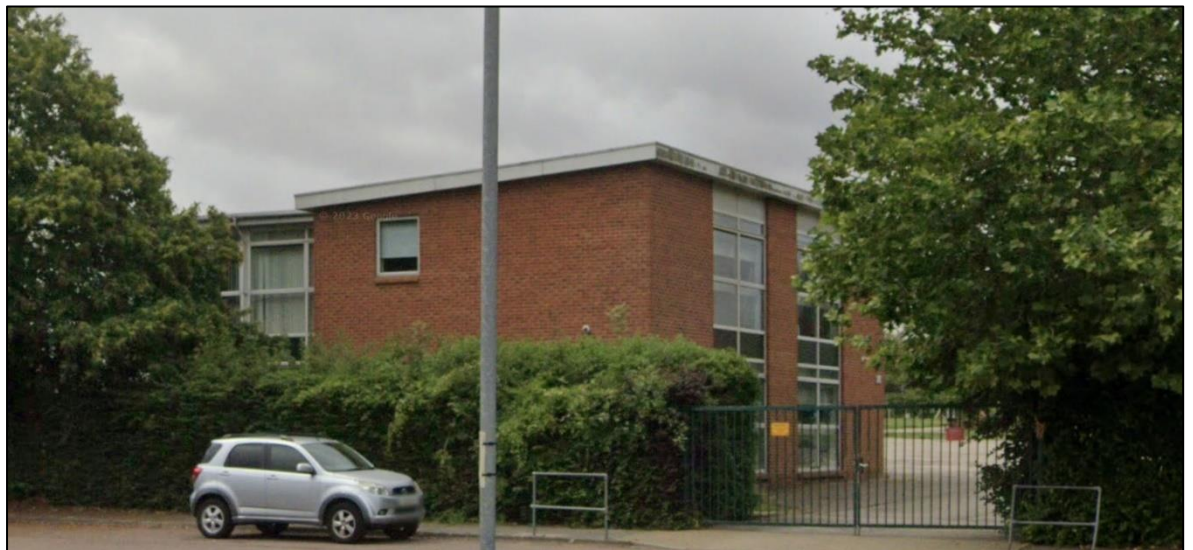
figure 72: Building Indicated as being Demolished
